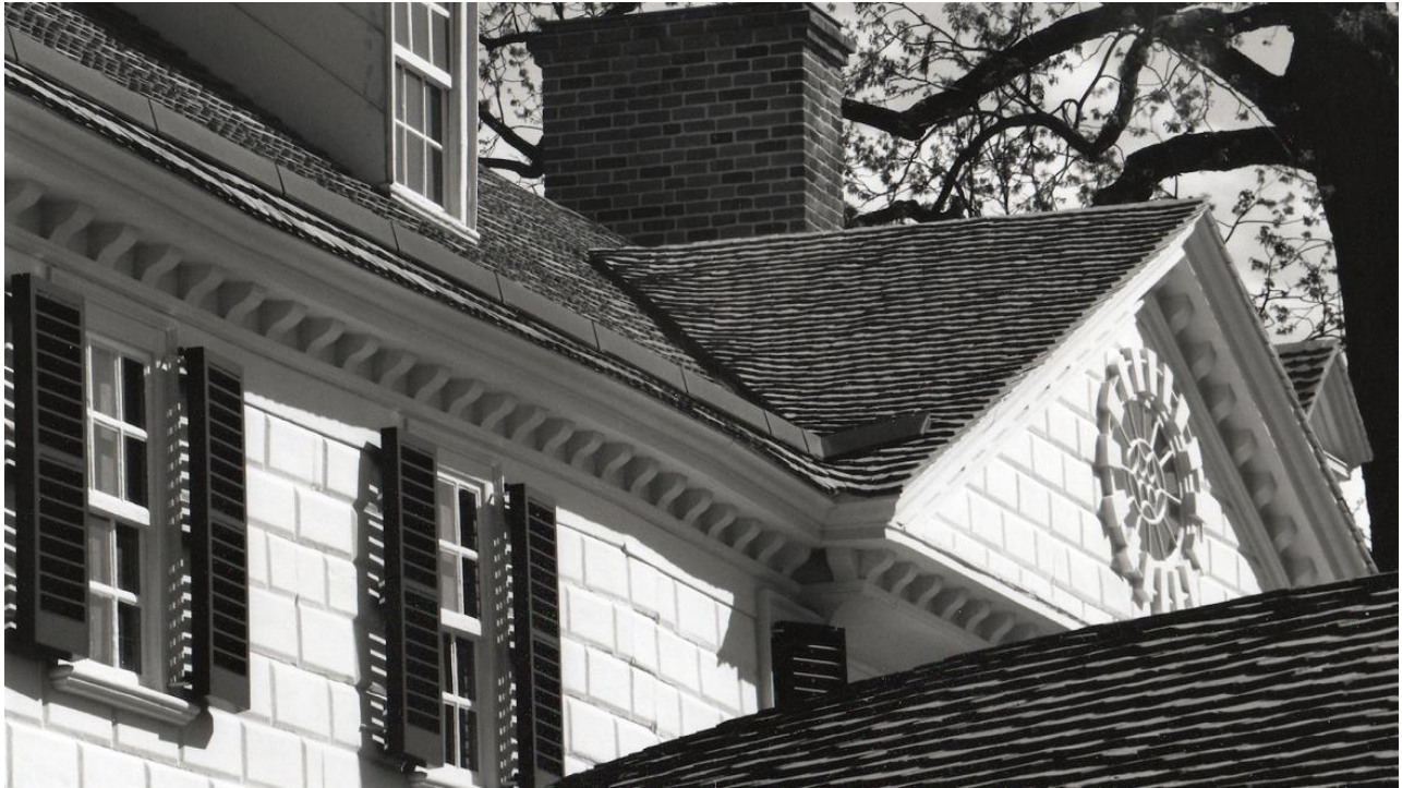
Architectural detail of Mount Vernon (Photo by Steve Ember)
